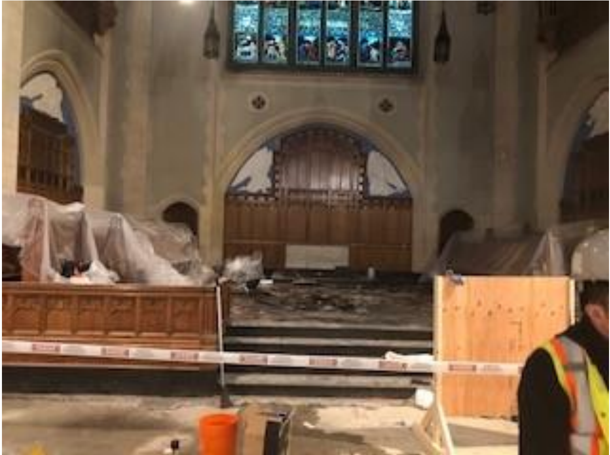
Chancel with flooring removed
