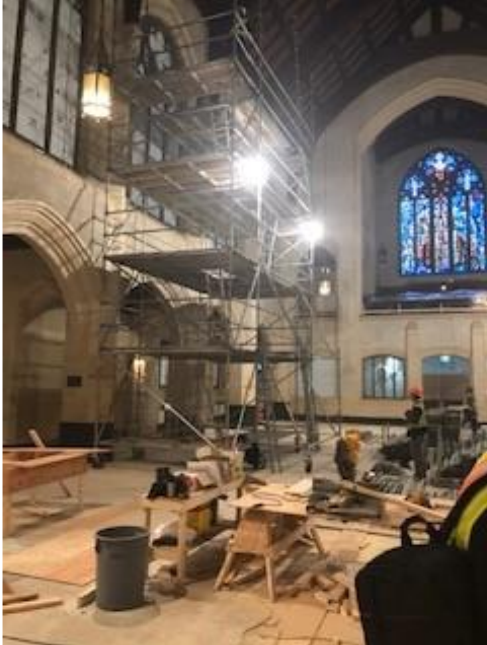
scaffolding in the sanctuary
