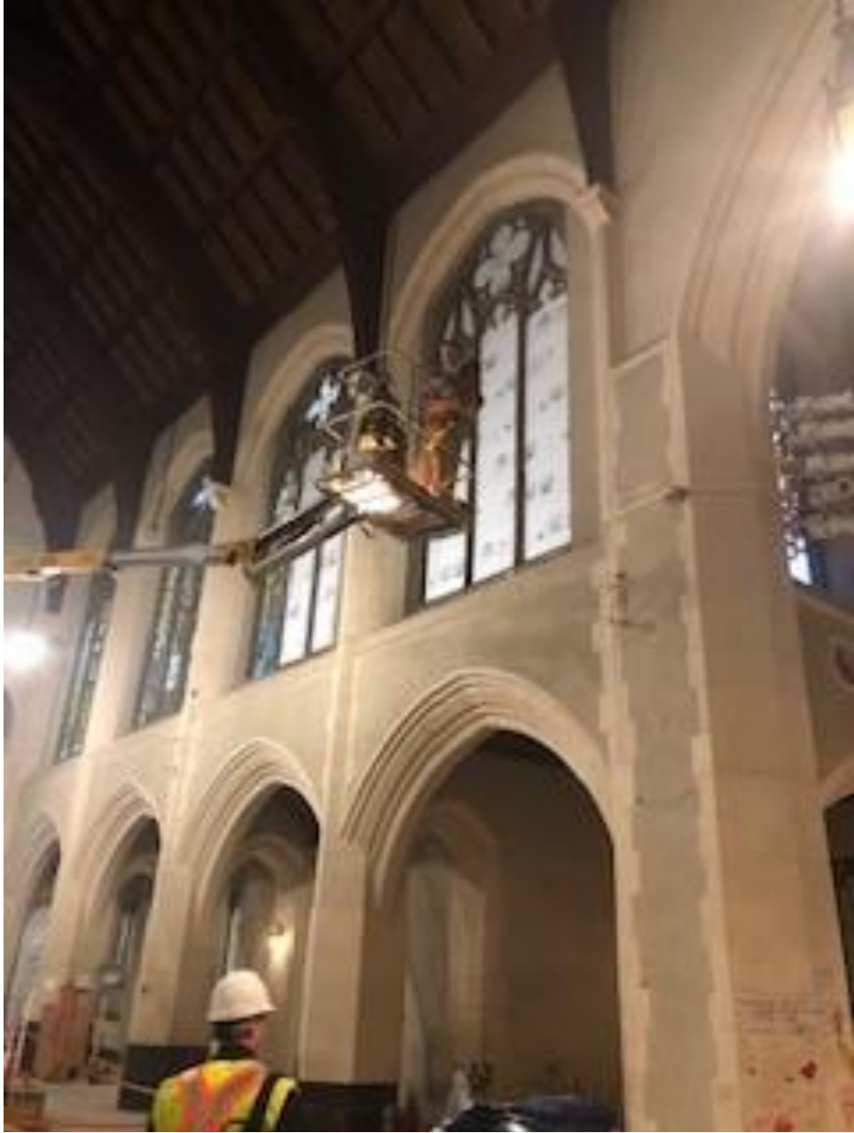
light fixtures being removed in the sanctuary
