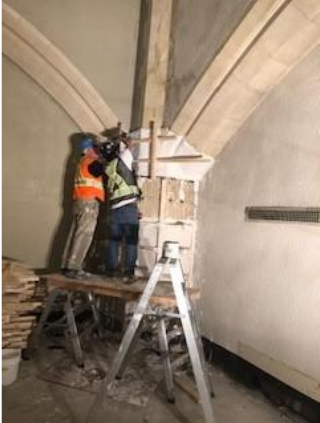
plaster moulds being made of the arches
