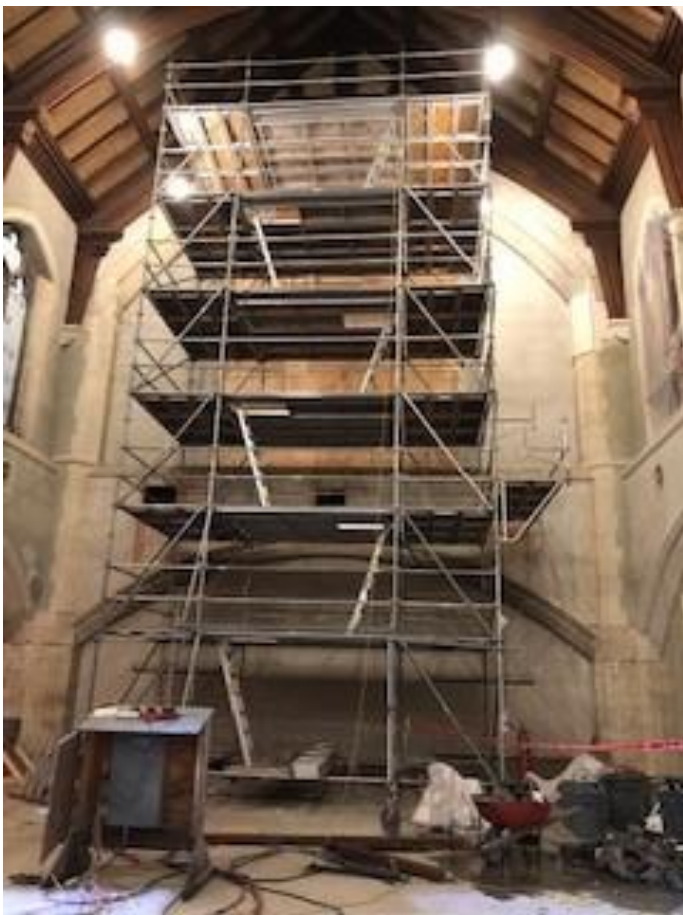
south transept window boarded up
