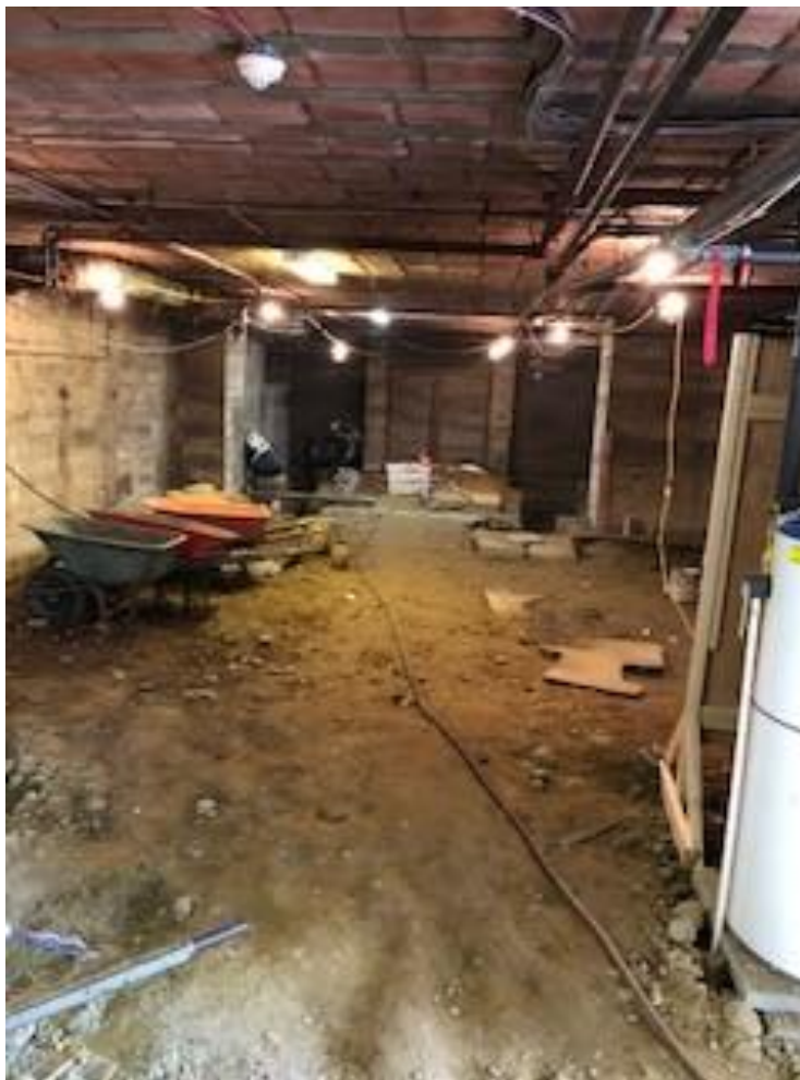
crypt, note the terracotta ceiling which supports the Narthex
