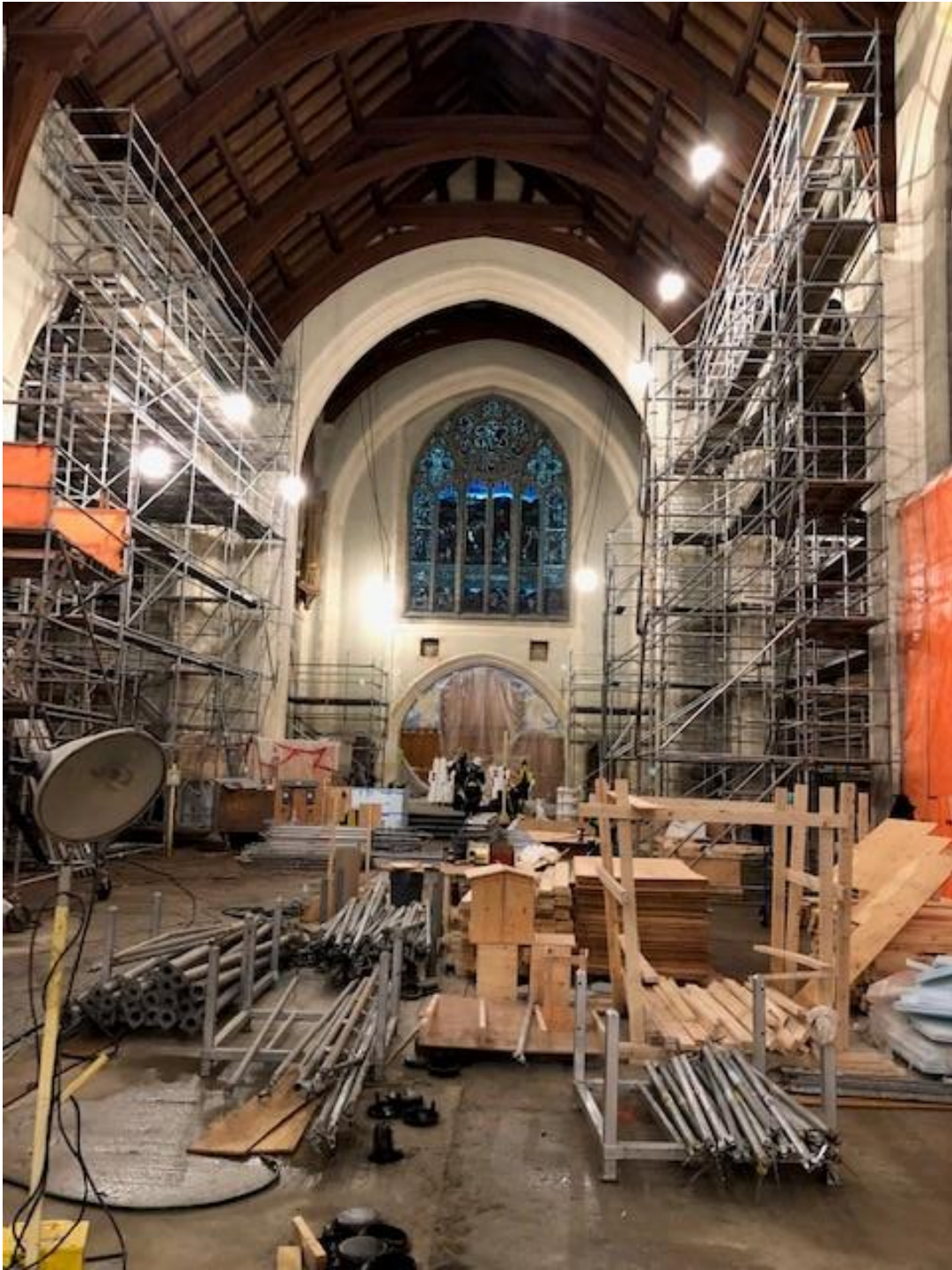
7 scaffolding to the ceiling
