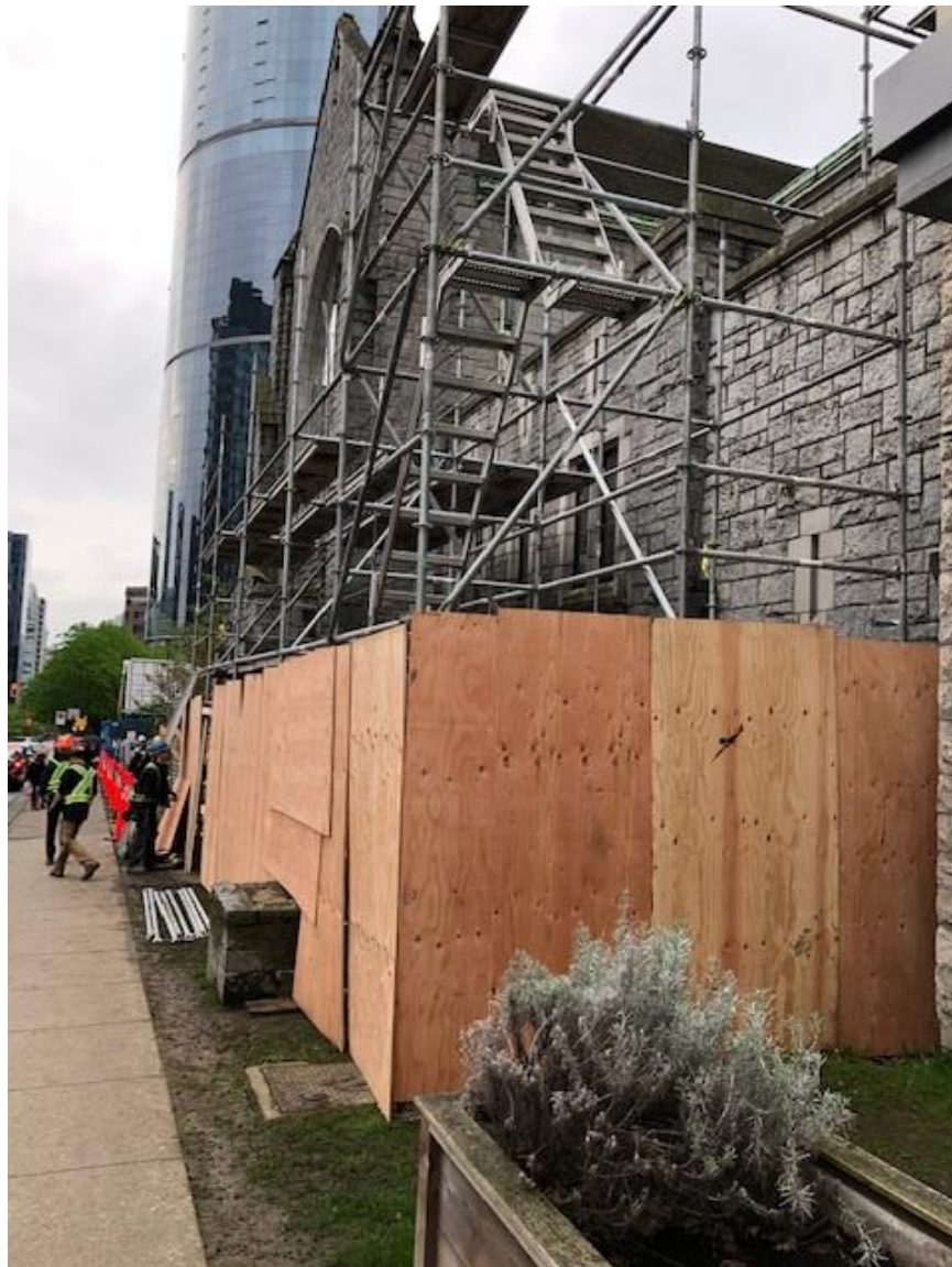
1 Scaffolding on Nelson St.
