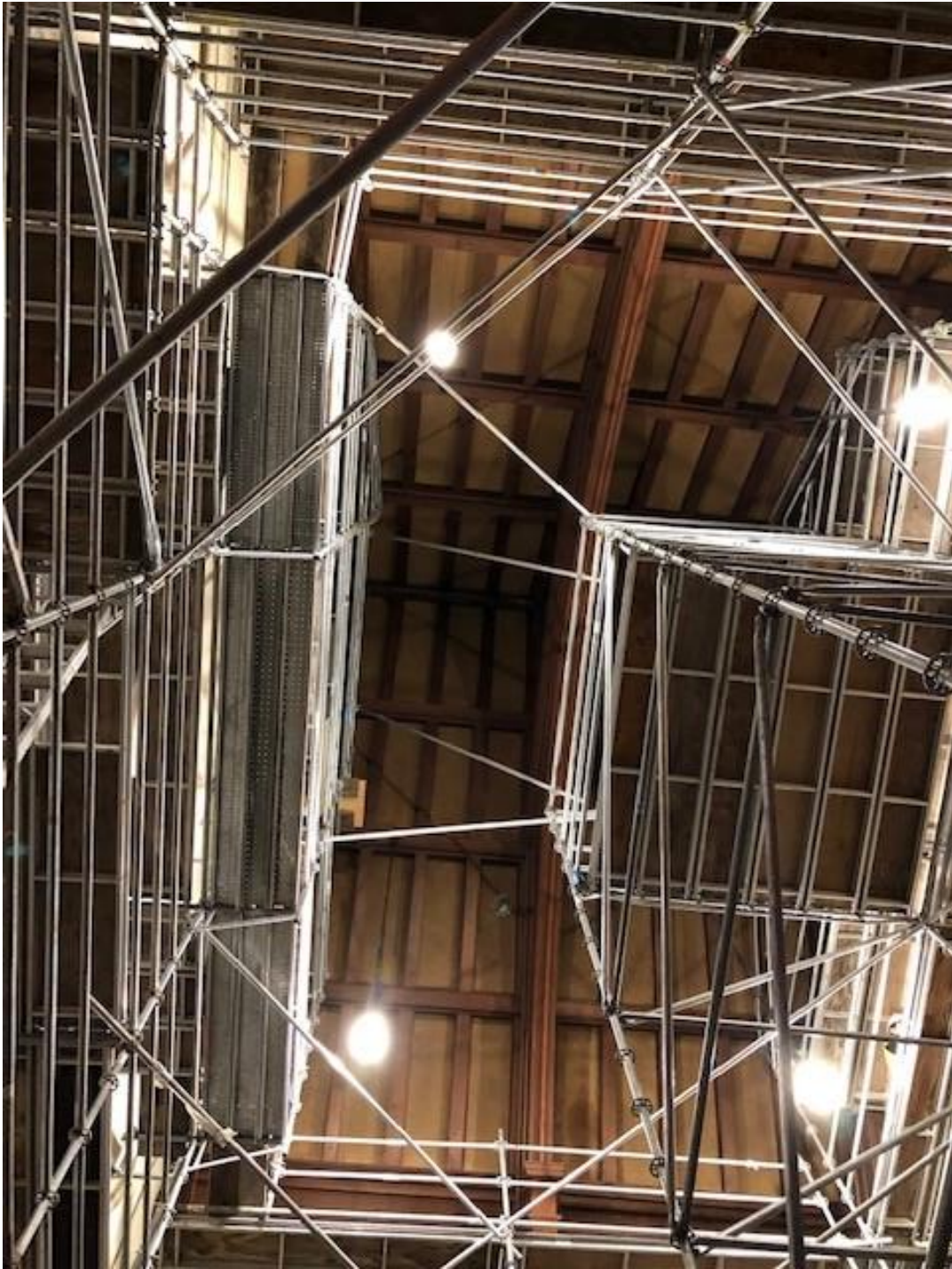
3 Scaffolding fills the whole transept, looking up at the ceiling.
