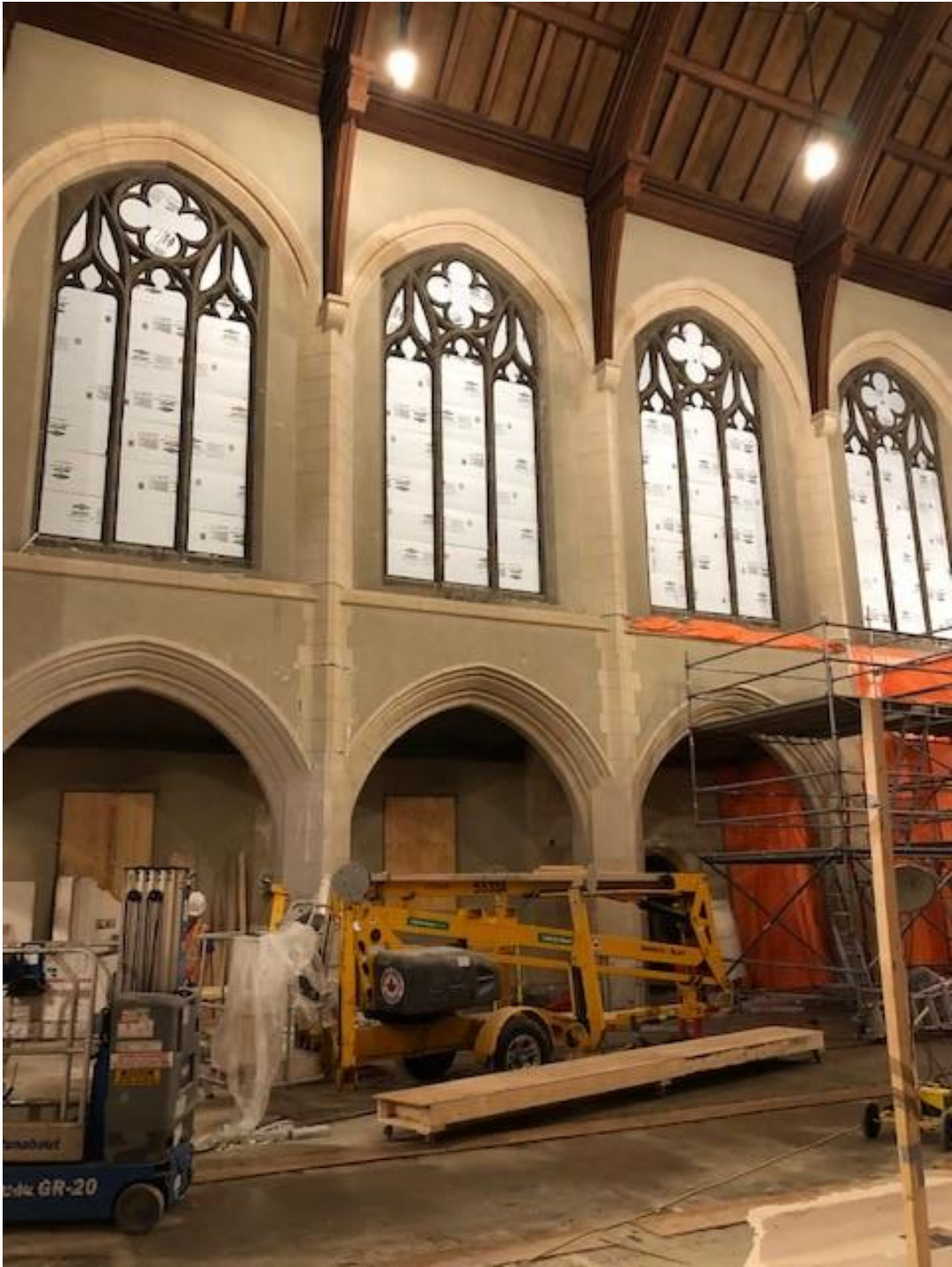
4 Stained glass windows hoarded
