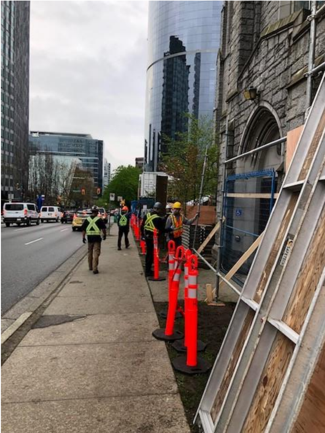
2 Pylons used to block a lane on Nelson St. and the sidewalk
