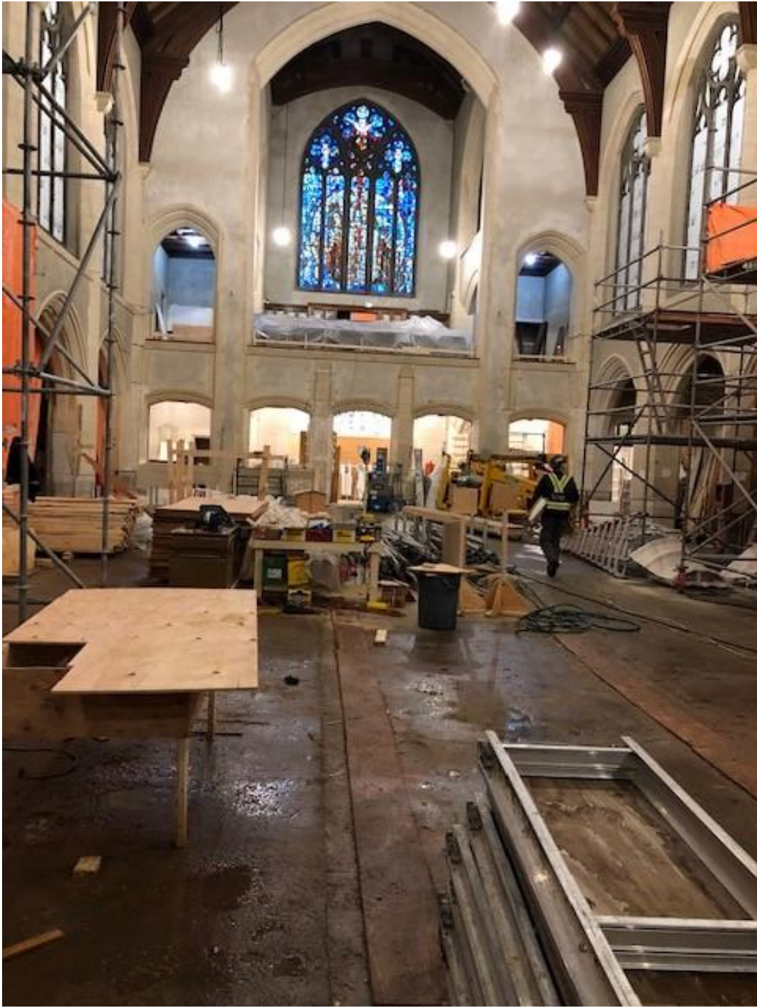
8 a lot of material and equipment in the sanctuary
