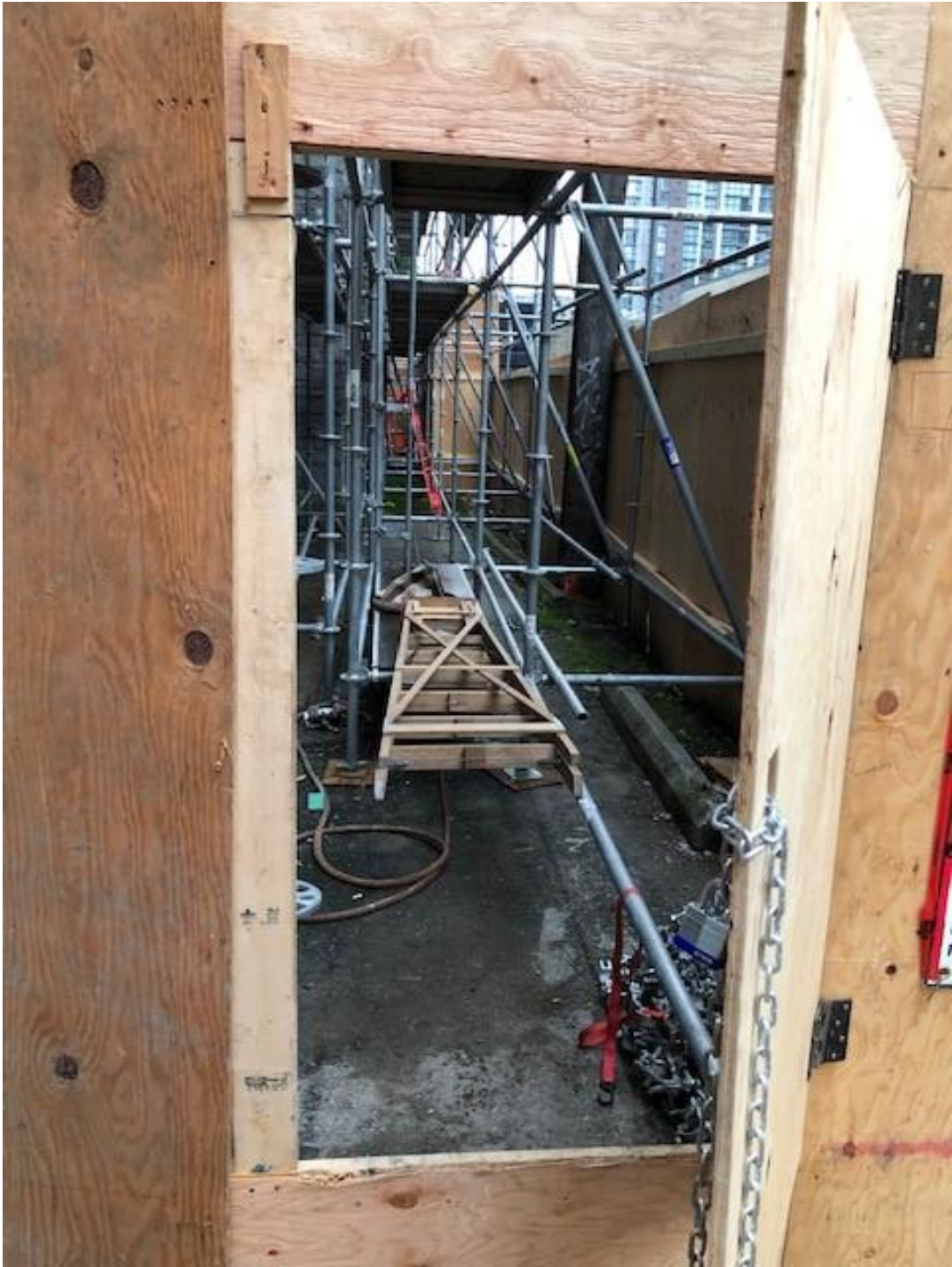
9 little door into scaffolding on exterior of the building
