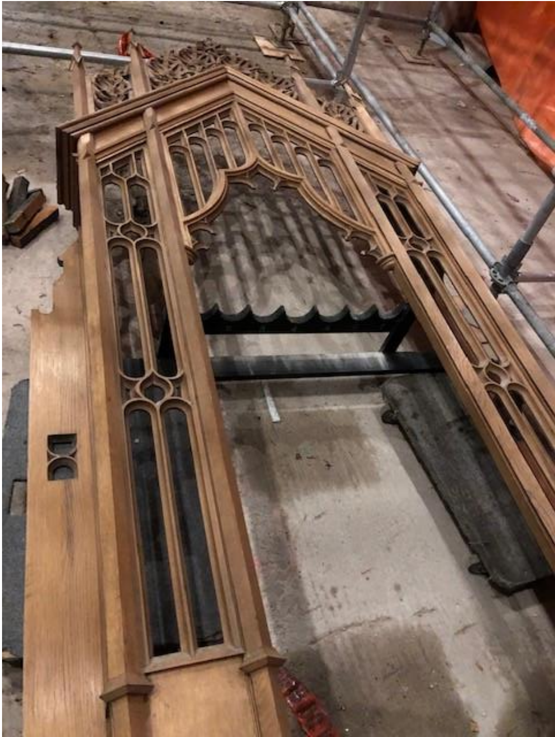
organ pipe facade removed and on floor
