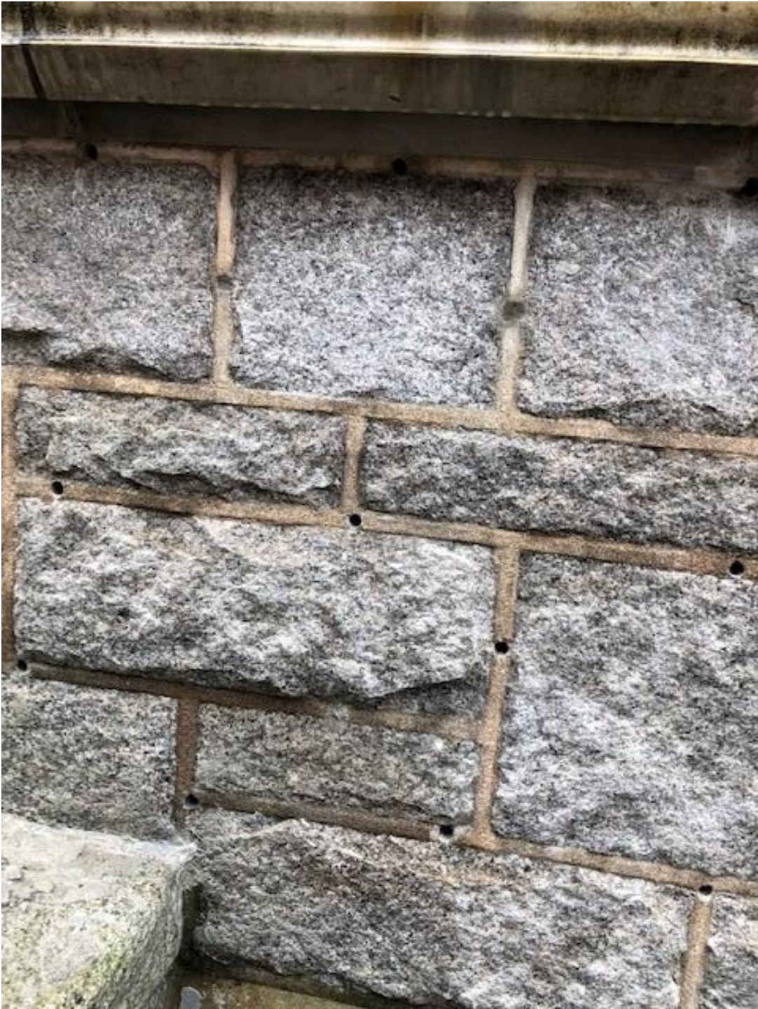
holes drilled into the exterior stone to determine how to anchor
