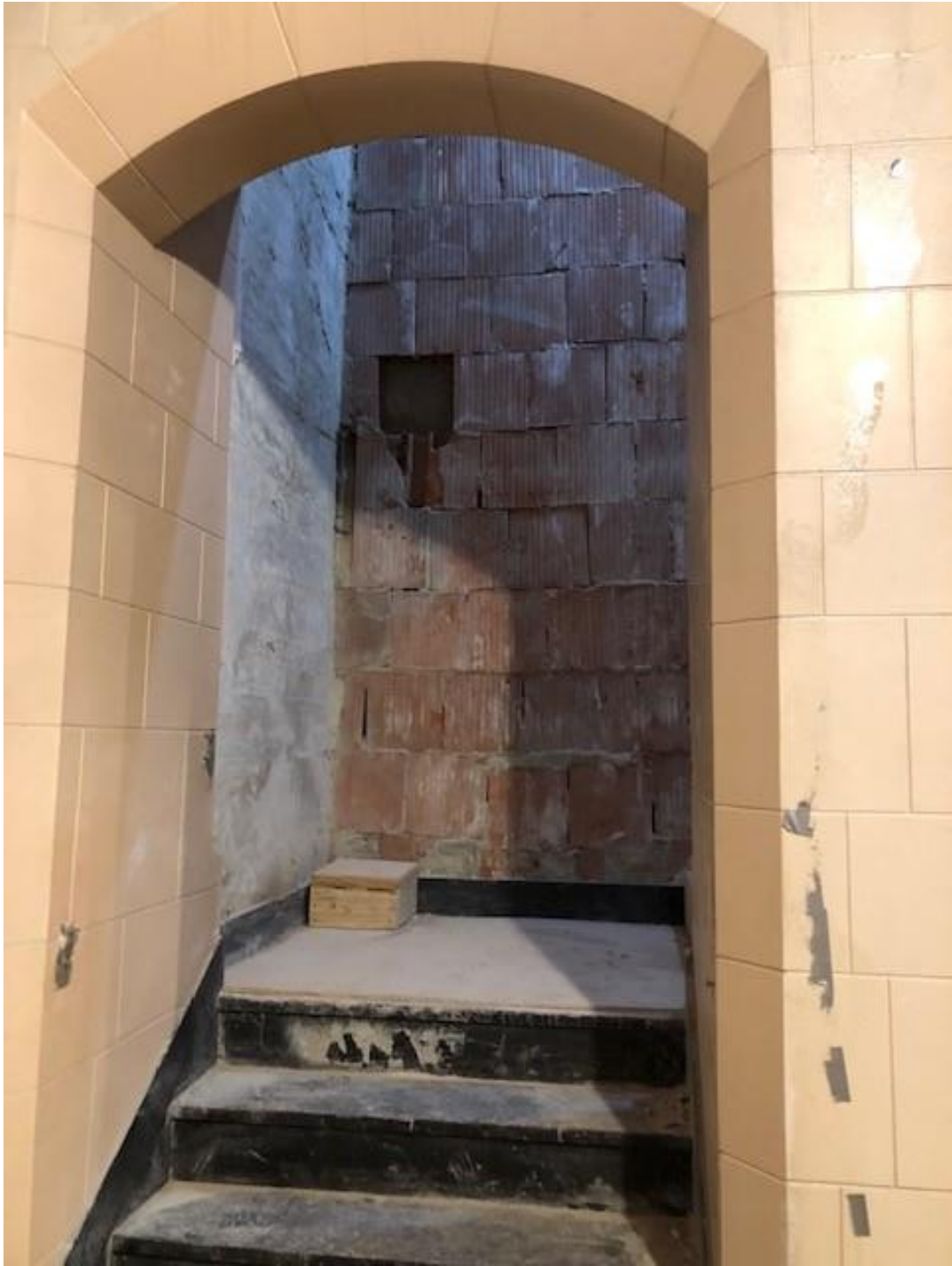
left stairwell to balcony, more terra cotta
