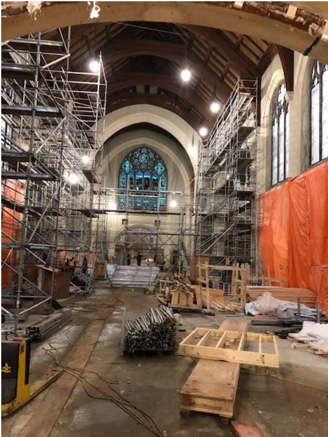
scaffolding, scaffolding everywhere
