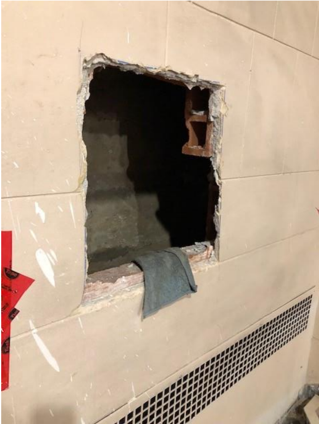
Narthex wall, plaster, terra cotta, then a big space until you reach the concrete
