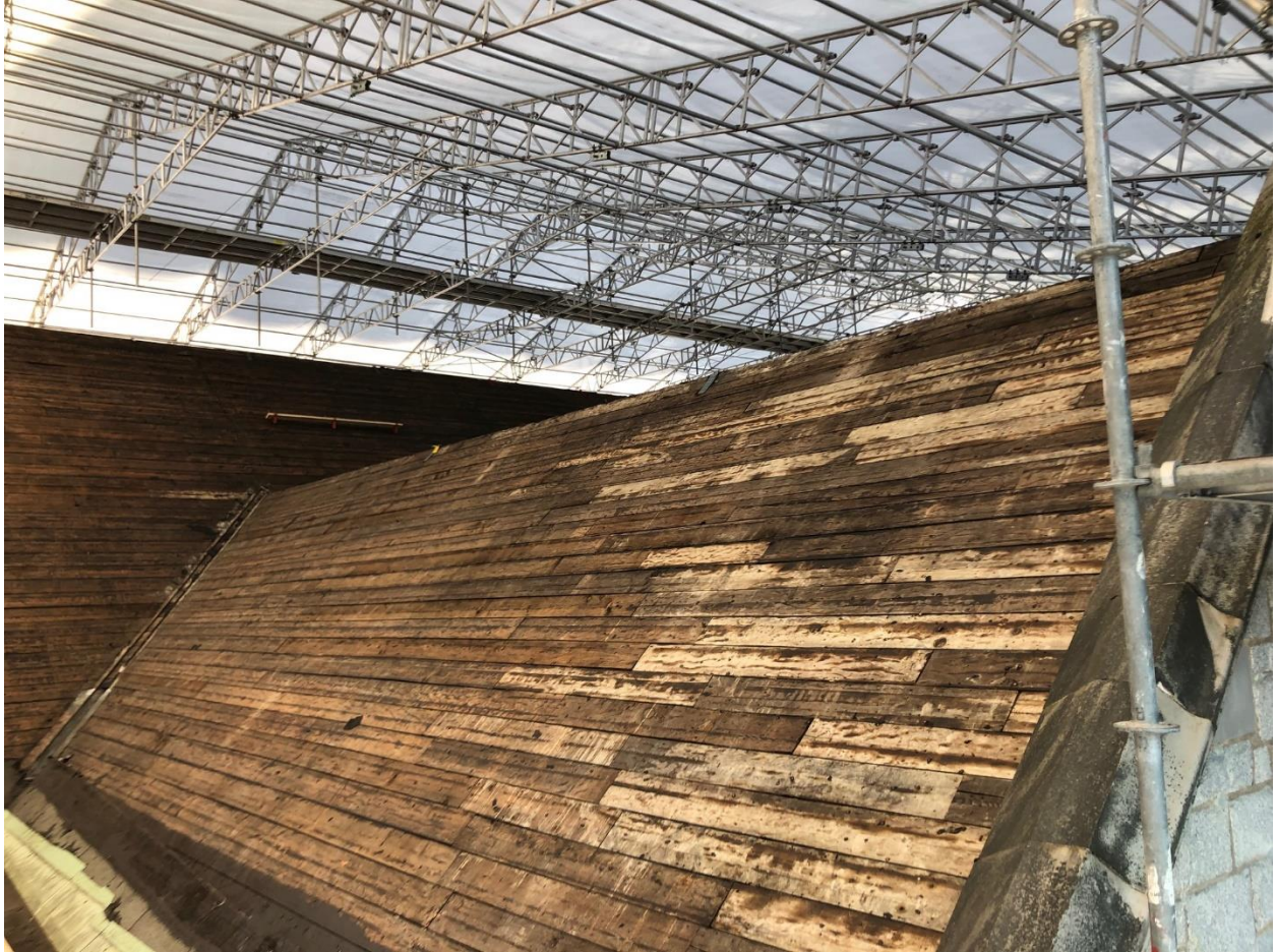
Asphalt roof removed
