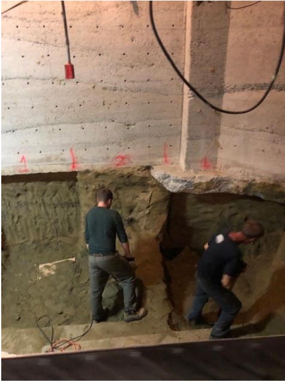
Digging for a new foundation for a shear wall on the sanctuary wall by the Ark room
