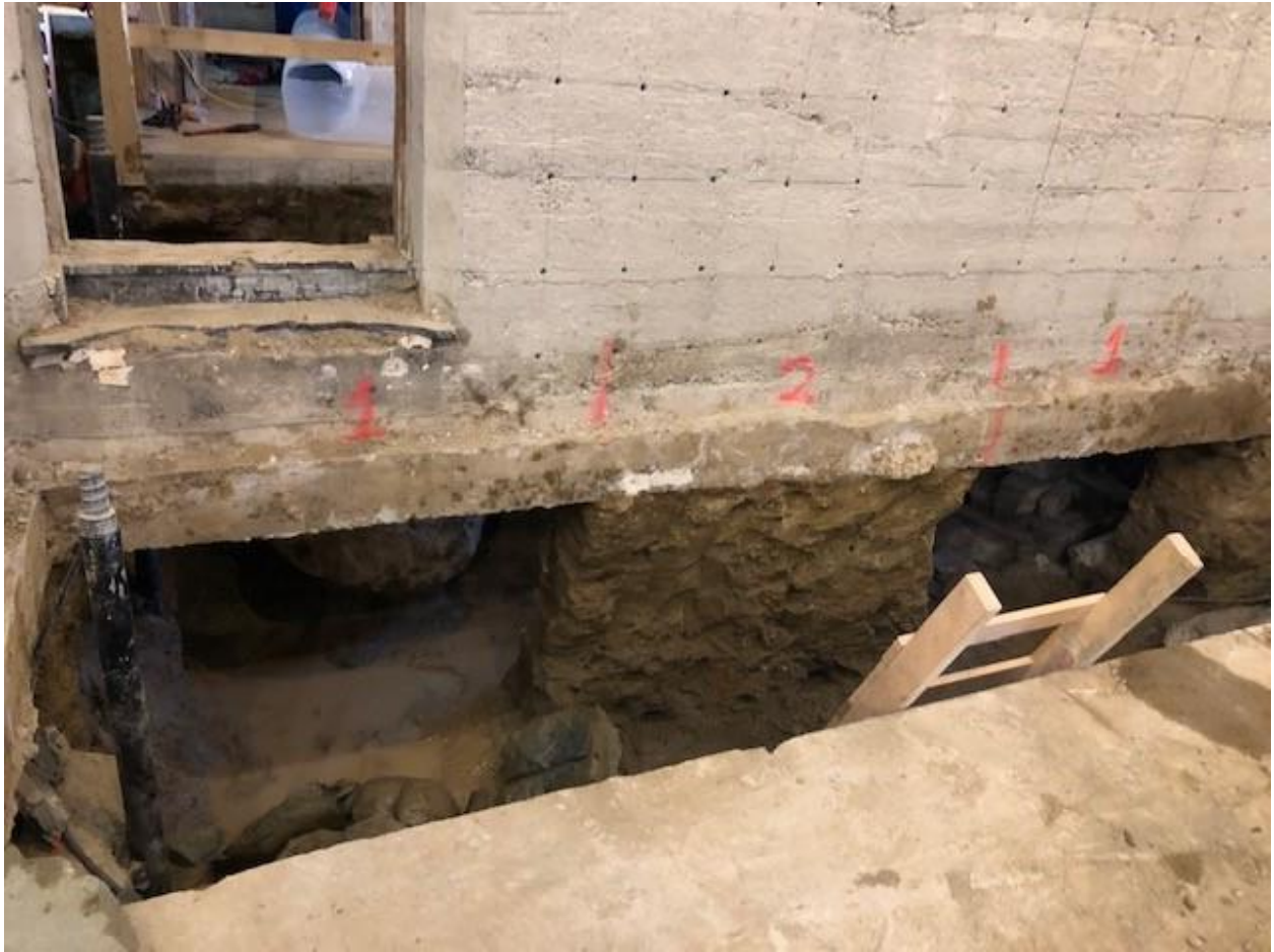
Digging under the Sanctuary wall by Marnie's room for the new foundation
