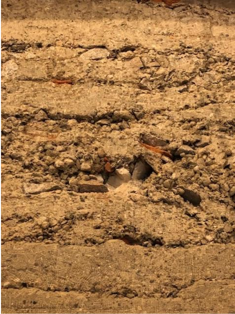
Original concrete wall with terra cotta
