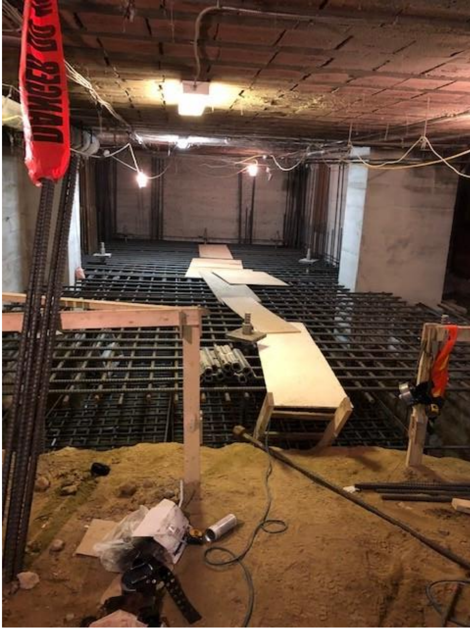
8 feet of rebar for the new foundation in the crypt
