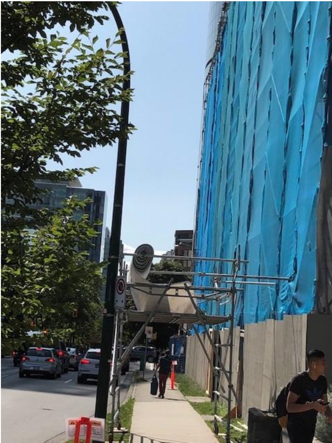
4 rolls of tarping for roof trusses
