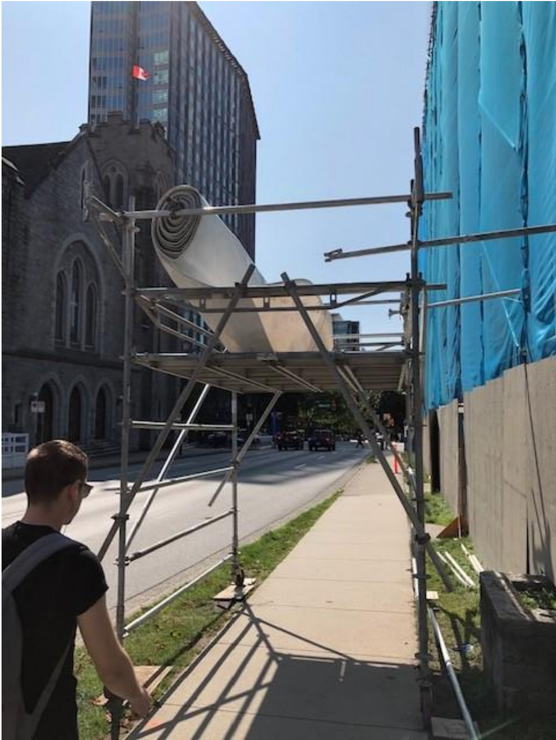
5 roof tarping on Nelson St.
