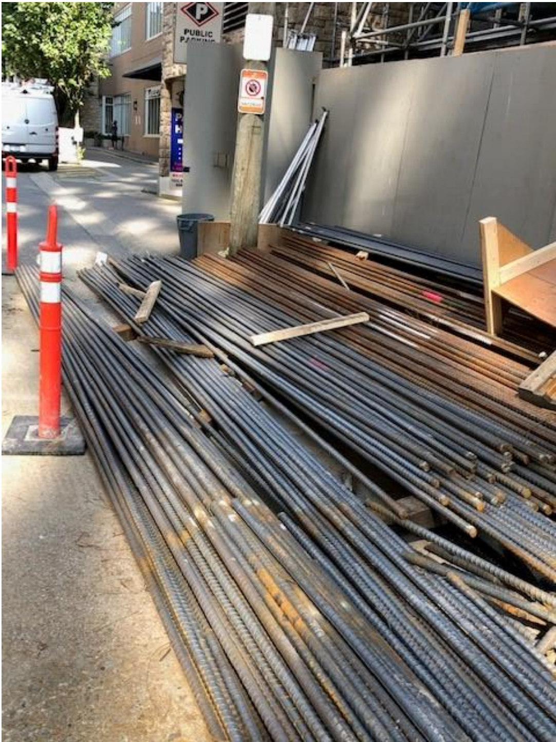
2 rebar for crypt
