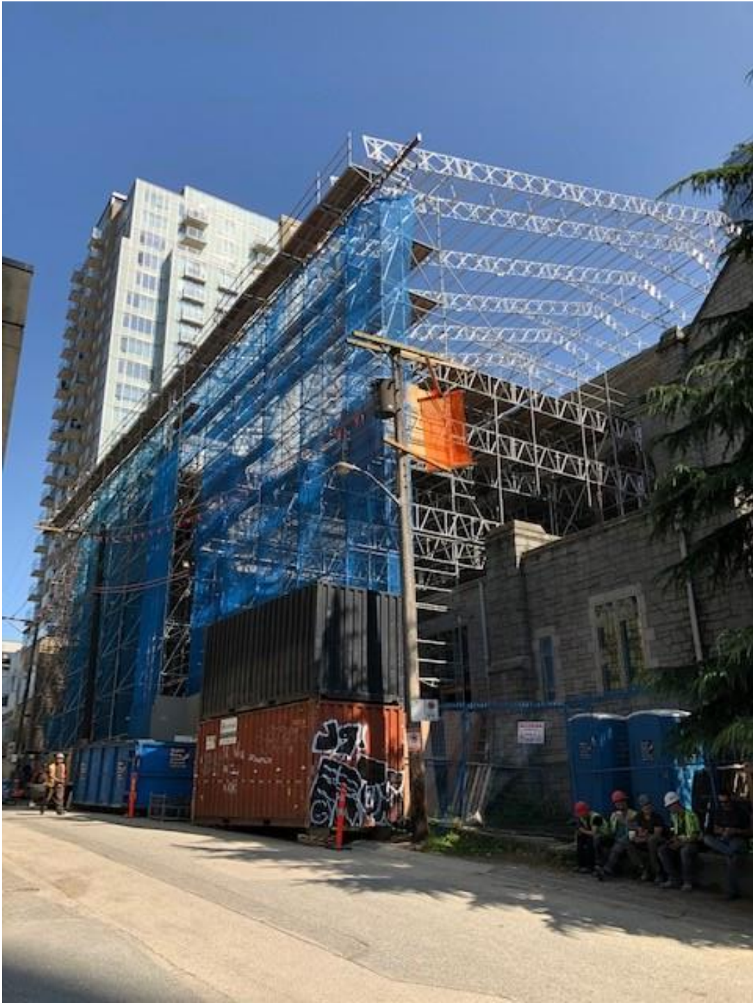
6 roof trusses from the lane
