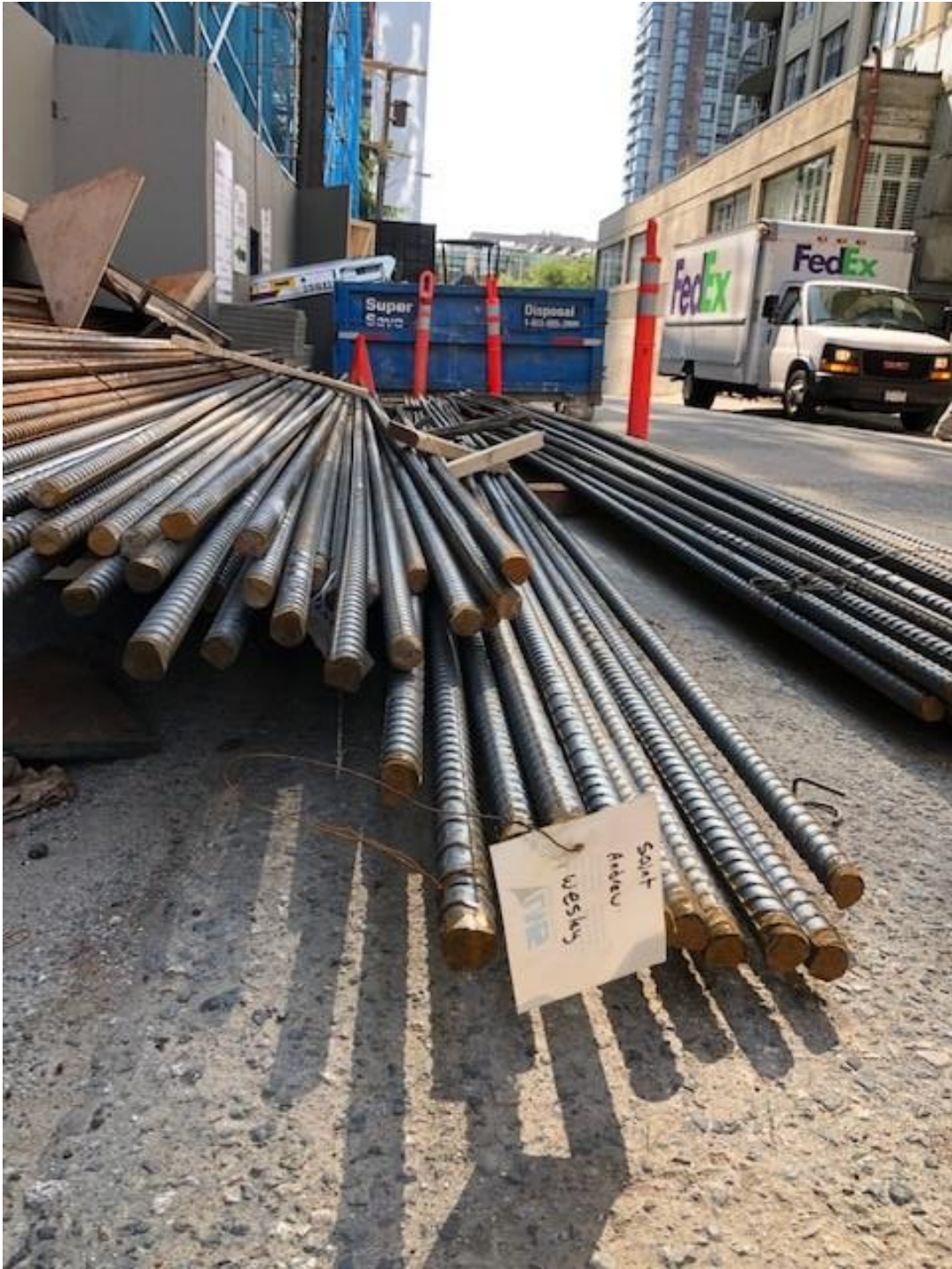
3 rebar for the crypt foundation
