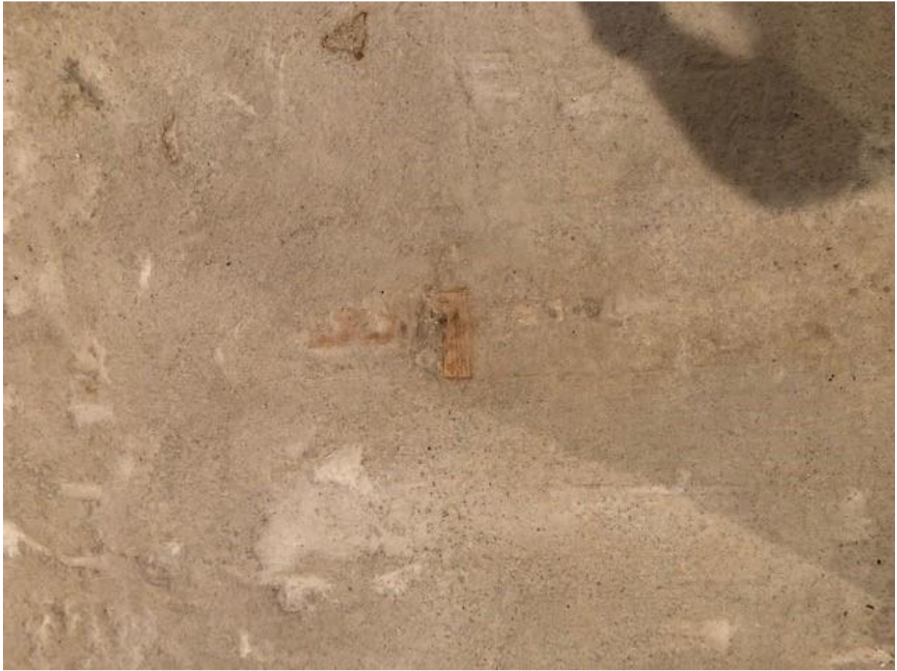
Wood in floor to screw in pews
