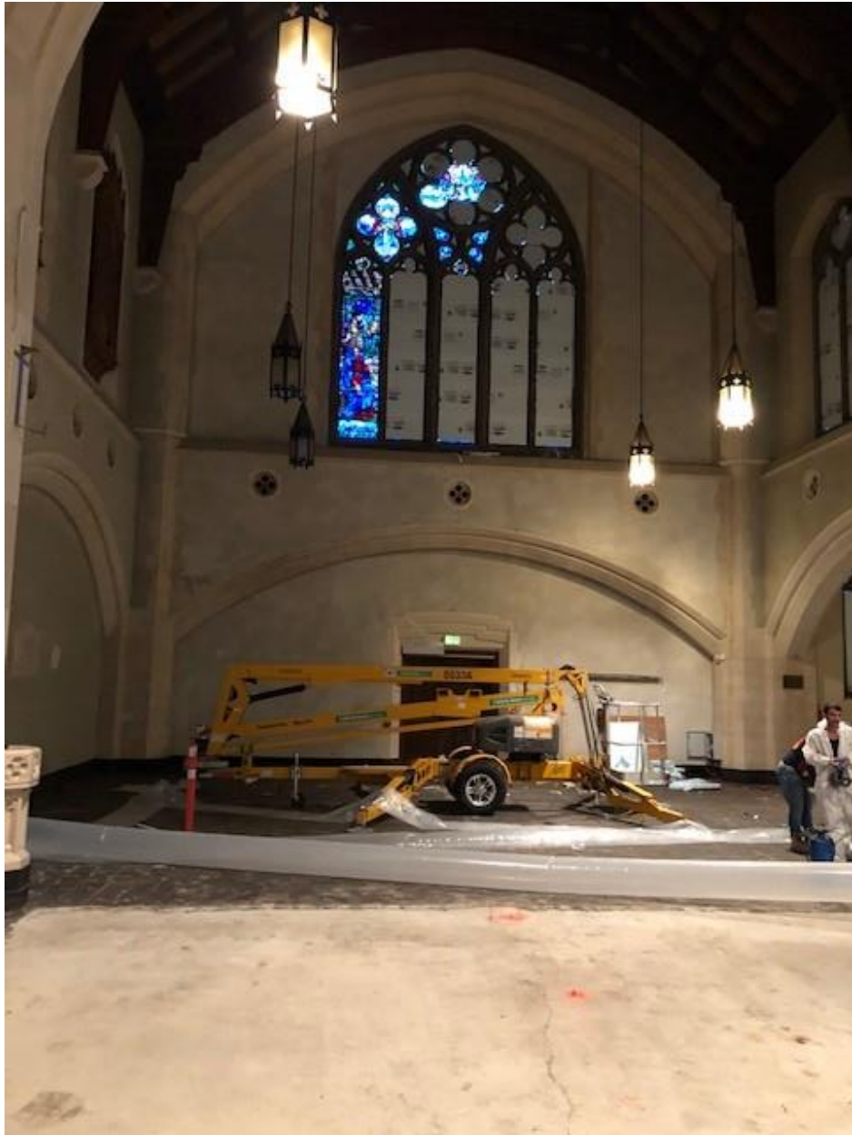
Hoarding North Transept
