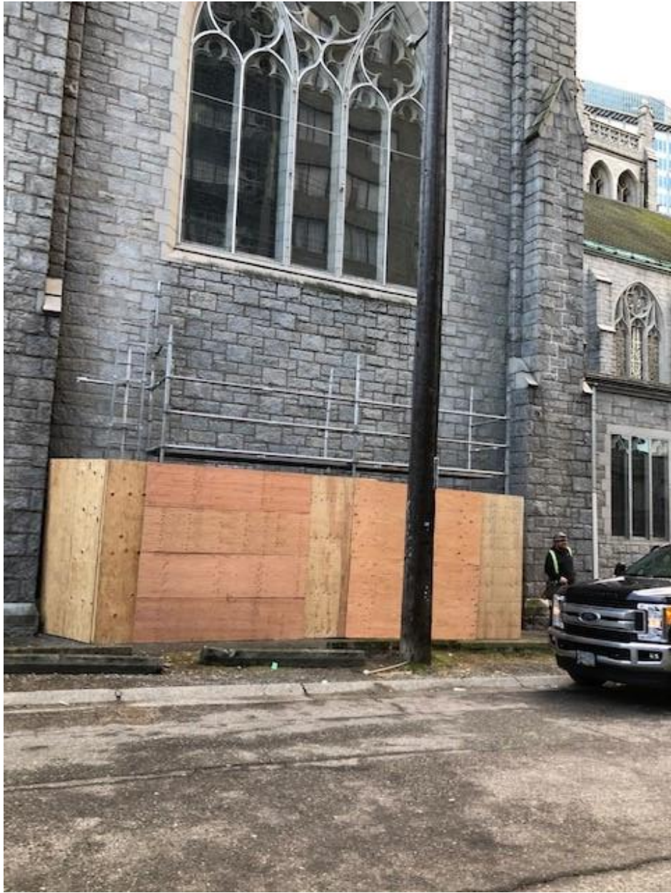
Scaffolding on the outside
